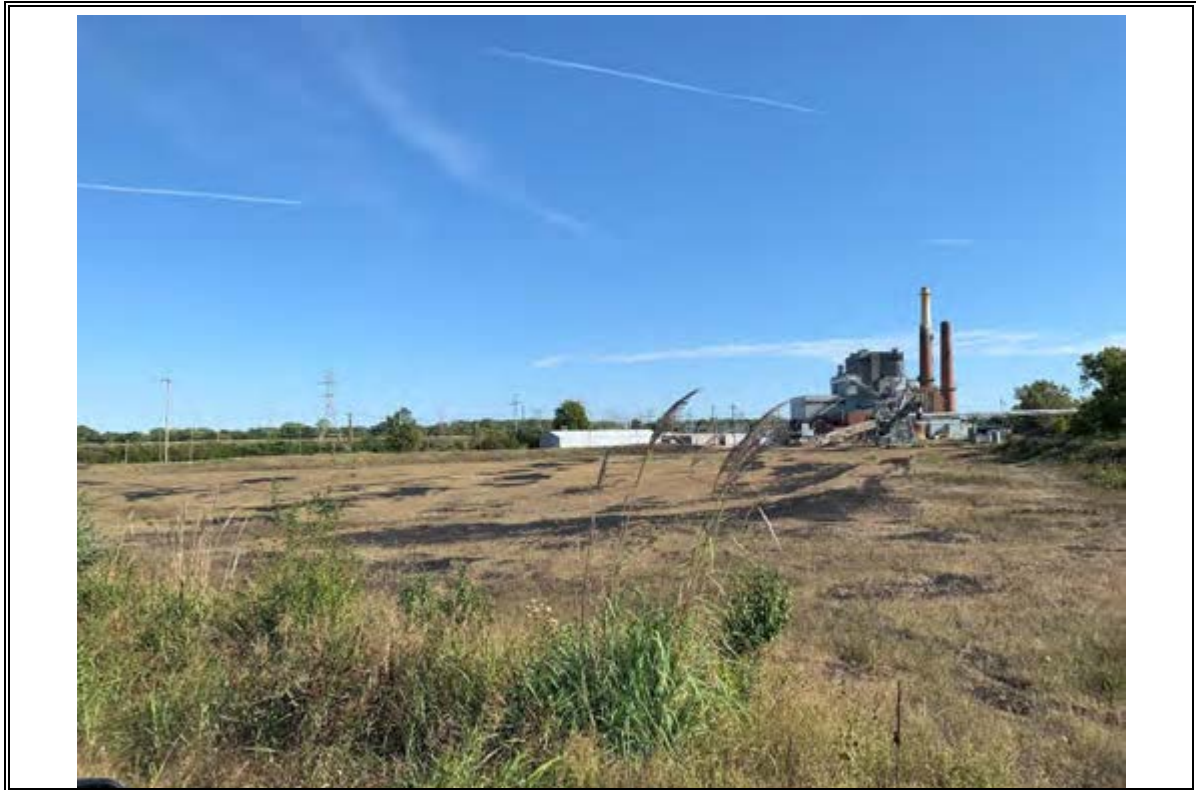
Photograph Number 15: Former coal Storage area west of the Power Plant. Facing East.
