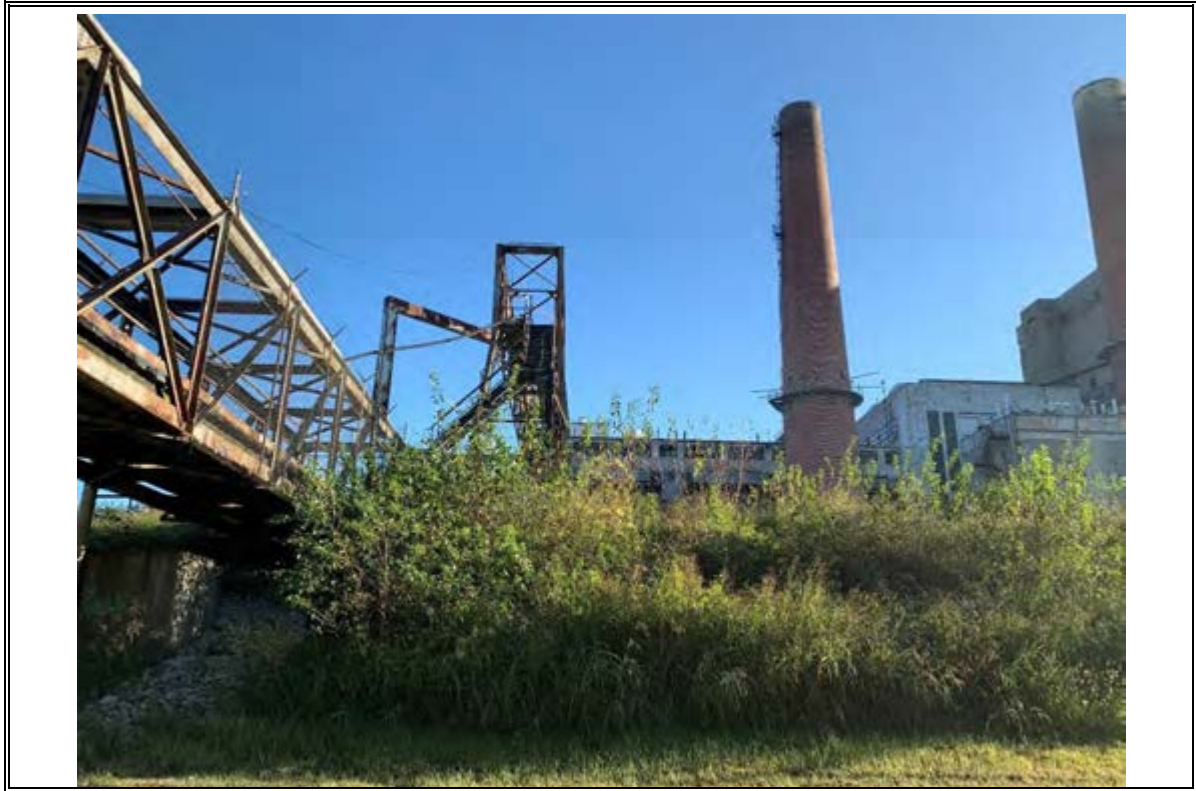
Photograph Number 27: View of extension's connection to the facility. Facing north.
