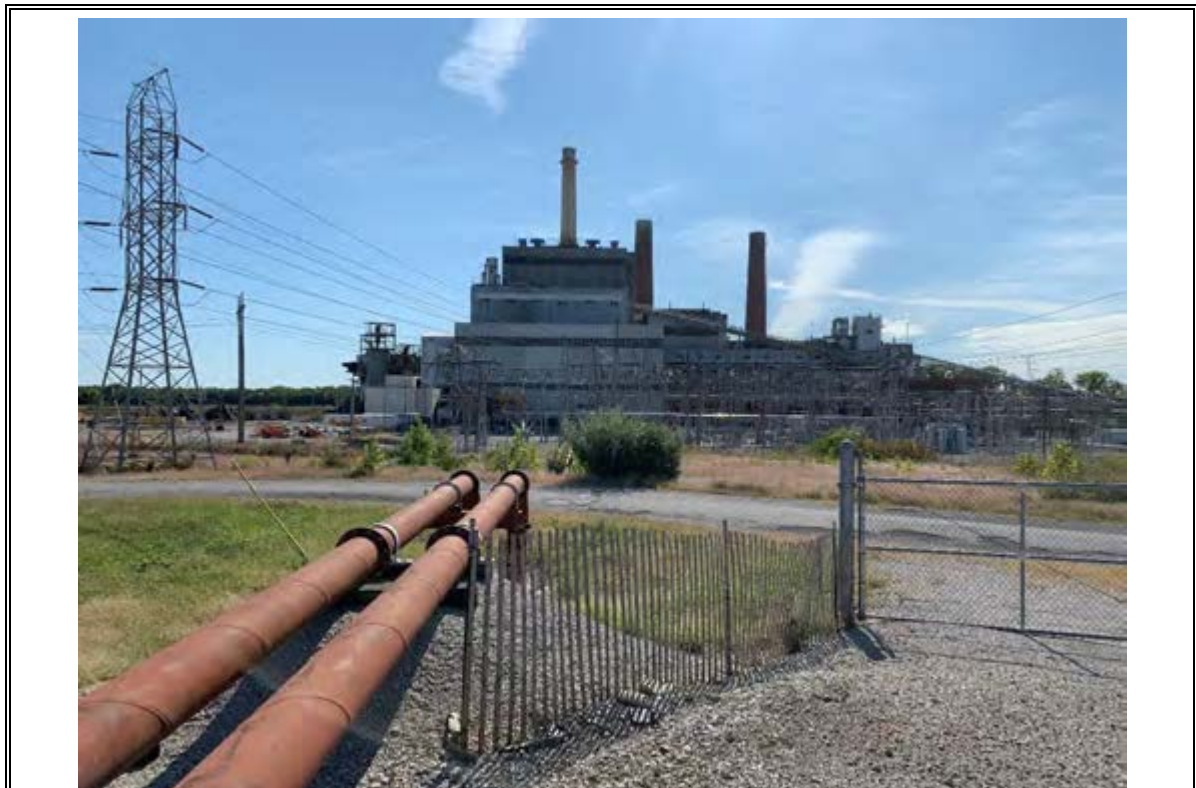
Photograph Number 12: Electrical substation and the former power plant. Facing South.
