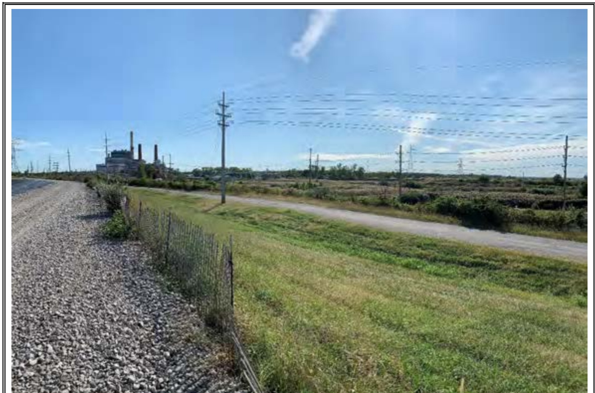
Photograph Number 6: View from East Ash pond dike, showing the upper access road, power plant, coal storage area, and West Ash pond. Facing southwest.
