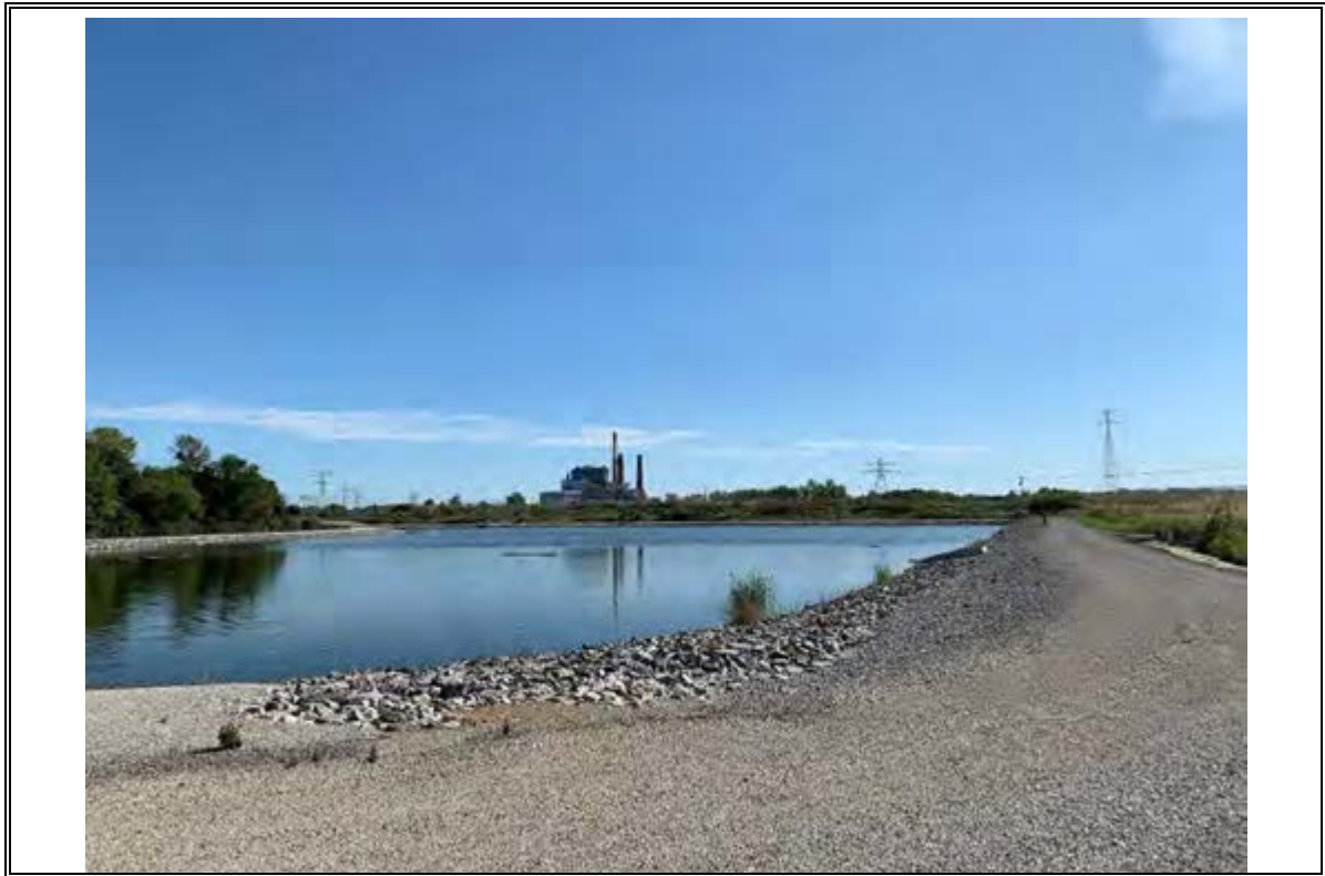
Photograph Number 25: View north across Pond 3.
