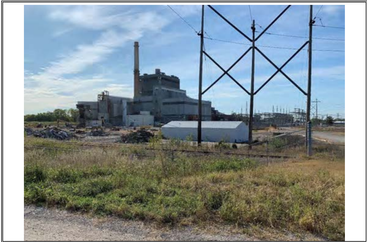
Photograph Number 3: View of power plant. Facing west.
