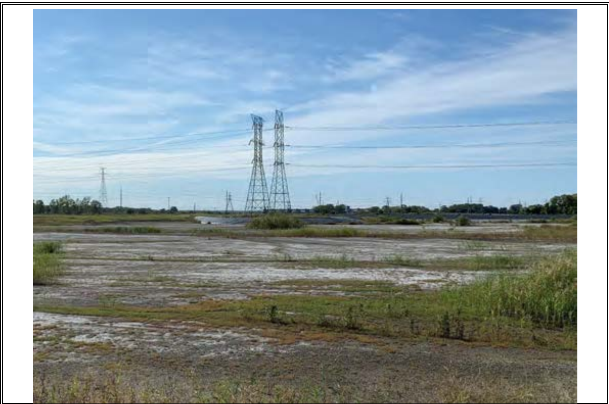
Photograph Number 10: The East Ash pond. Facing west.
