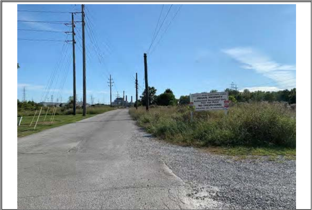
Photograph Number 1: North entrance to the facility. Facing south.
