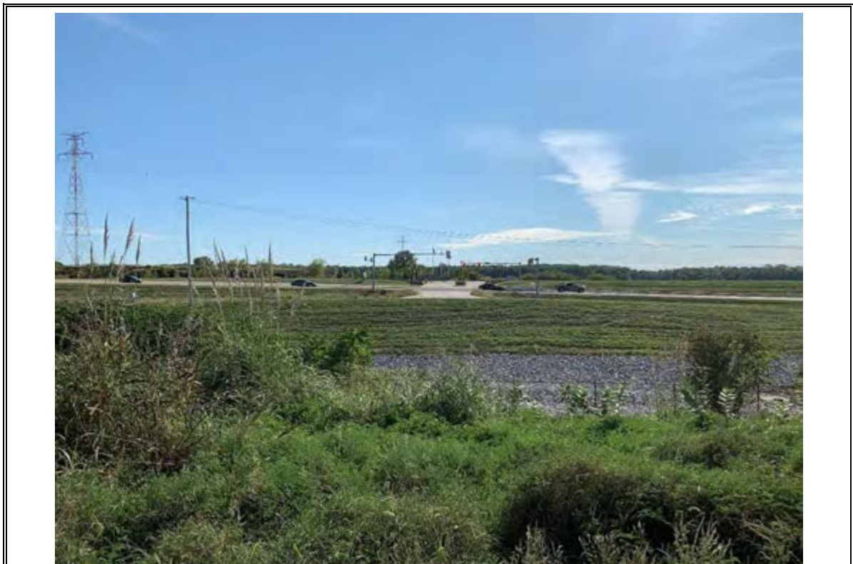
Photograph Number 16: Continuation of the levee along the south property boundary as well as IL route 143 and the Mississippi River levee.
